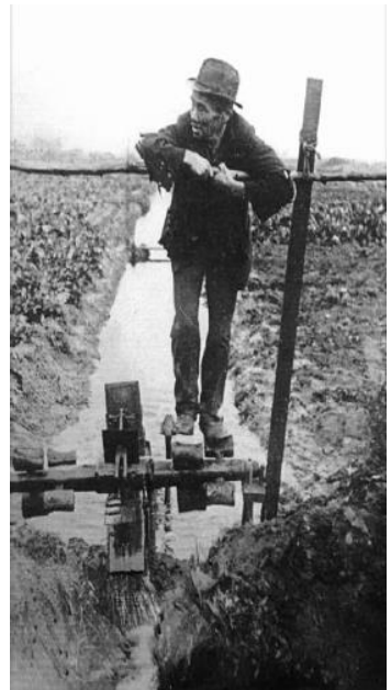
Foot powered, Chinese water pump used on the goldmining races
